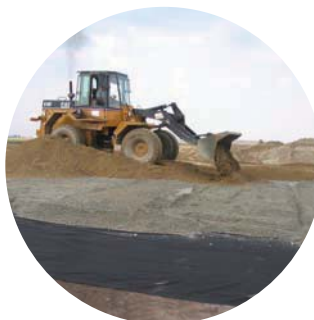
Middle: Axminster carpet with Bonar backing yarn. Right: Bontec SG 36/40 woven textiles for a pipeline project. Grijpskerk-Wurkum, The Netherlands.
